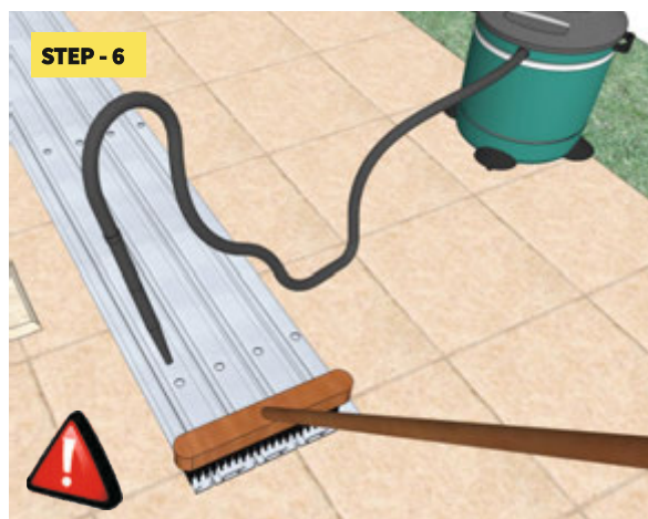
STEP - 6 Important to clean the rails of dirt, the best way is to use vacuum cleaner and sweep carefully.
