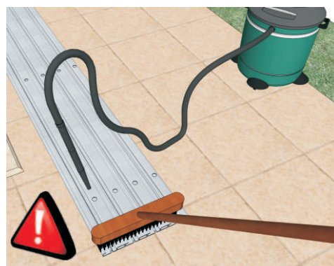
Important to clean the rails of dirt, the best way is to use vacuum cleaner and sweep carefully.
